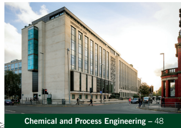
Chemical and Process Engineering – 48
