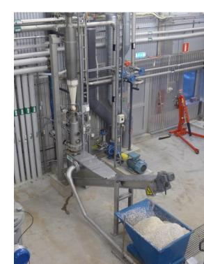
The slurry is dewatered and the residue compressed as a biofuel
